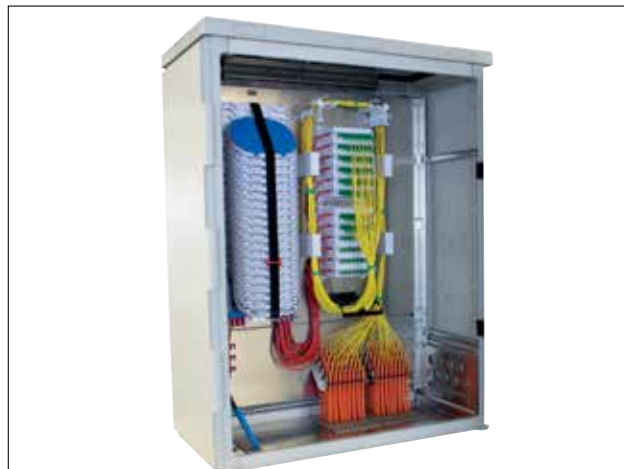
Point of Connection (door not shown)
