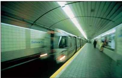
Tunnels a common application.
